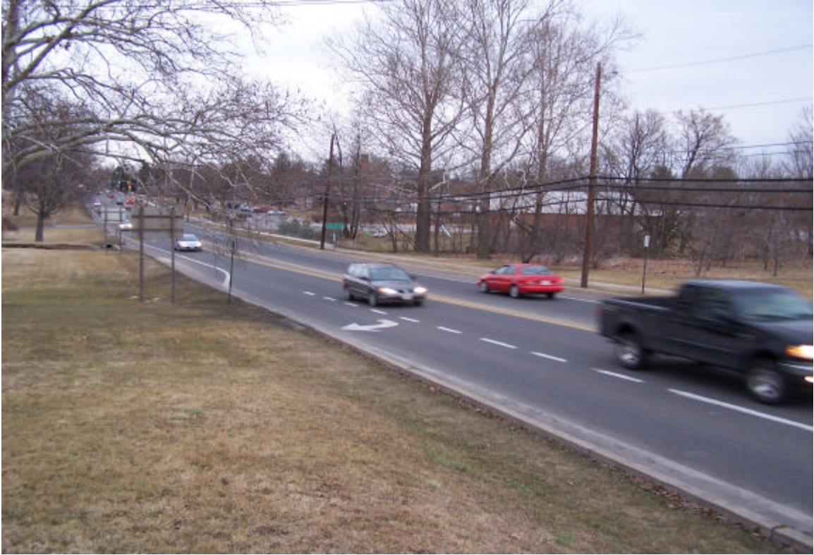
Picture 9 – Southbound Pennsylvania Avenue approaching Haven Road
