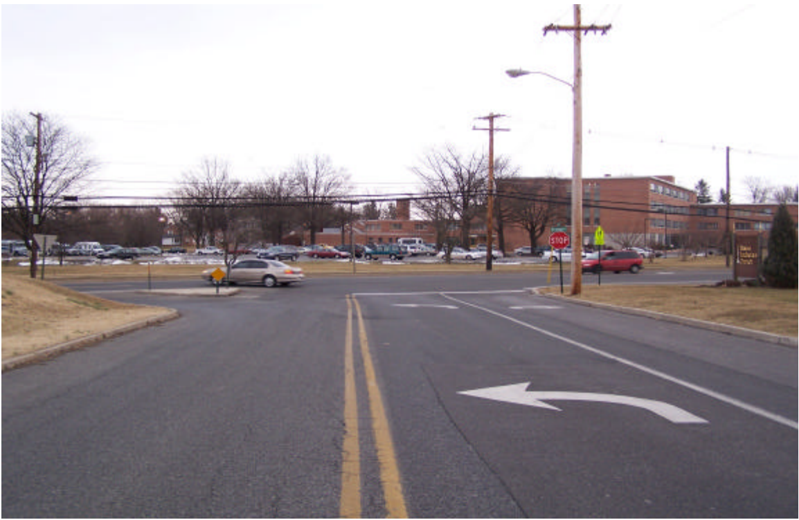
Picture 5 – Eastbound Haven Road approaching Pennsylvania Avenue
