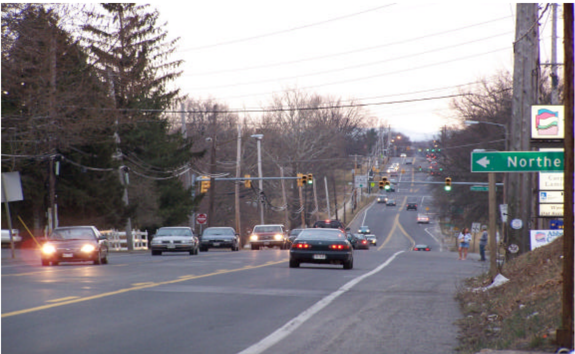
Picture 4 – Southbound Pennsylvania Avenue approaching Northern Avenue
